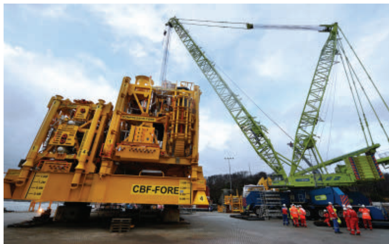
The Åsgard subsea compressor, shown here prior to installation in December 2014, is now the first plant to operate on the seafloor, rather than onshore or on a platform. (Courtesy Harald Pettersen, Statoil)
