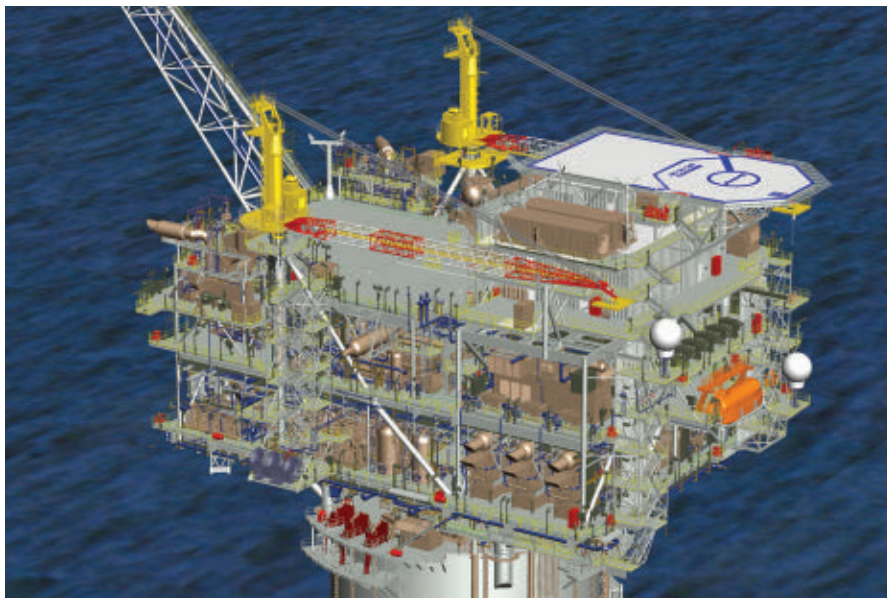
The Heidelberg field is located in the US Gulf of Mexico, at a water depth of 5,310 ft (1,620 m). (Courtesy Wood Group Mustang)
