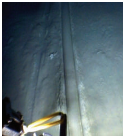
Export line impacted by blockage. (Photos courtesy Reaching Ultra)
