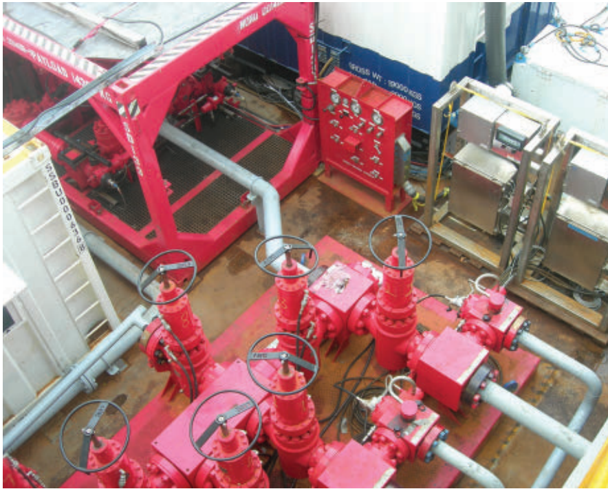
An MPD riser stack, equipped with a deepwater RCD and an annular isolation device, in mid-deployment.
